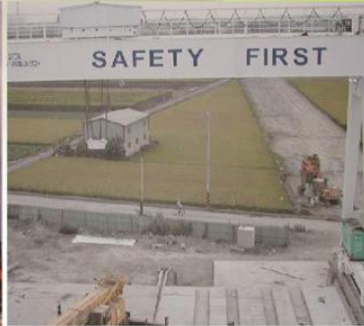
2001 Taiwan High Speed Rail 100 tons gantry crane
