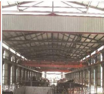
2001 Taiwan High Speed Rail mobile plant
