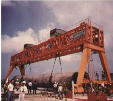
1988 Bali, Taipei 200 tons crane project
